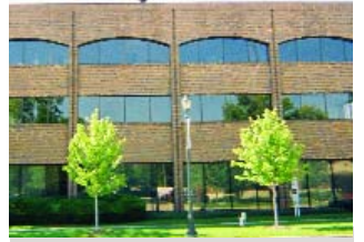
Northfield Satellite Office
